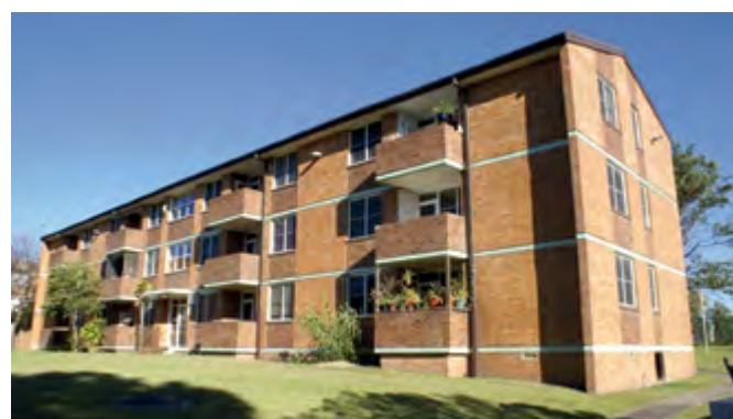
Bilga Crescent housing estate, Malabar (photo by Anthony Markakis)
